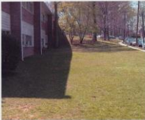
The front yard (BEFORE)
