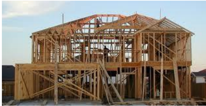
Wood Frame Construction
